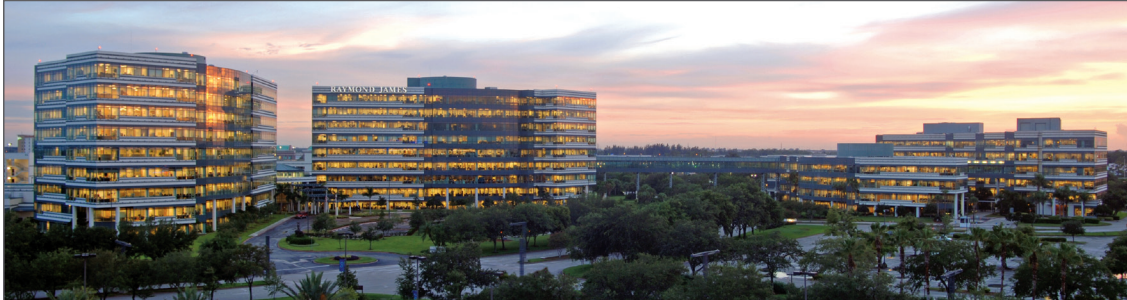
Raymond James International Headquarters in St. Petersburg, Florida
